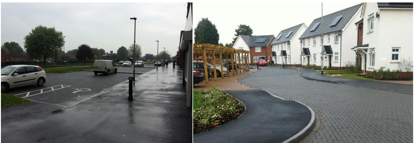
Figure 7-2 Award winning permeable paving sites at Central Avenue and Fleetwood Crescent
