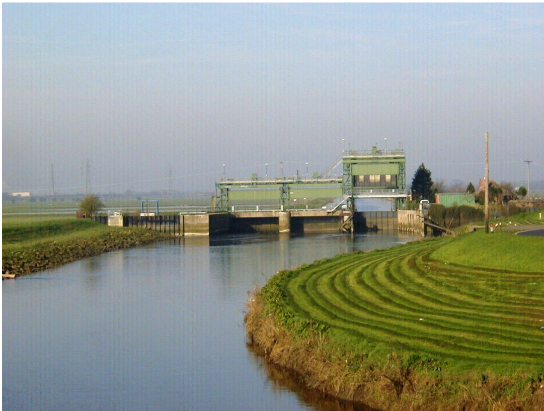
Figure 5-3: Dog in the Doublet sluice when the tide is not so high. Source: Environment Agency.
